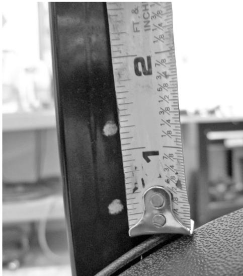
Mark Mounting Holes And Drill With A 9/32" Bit
